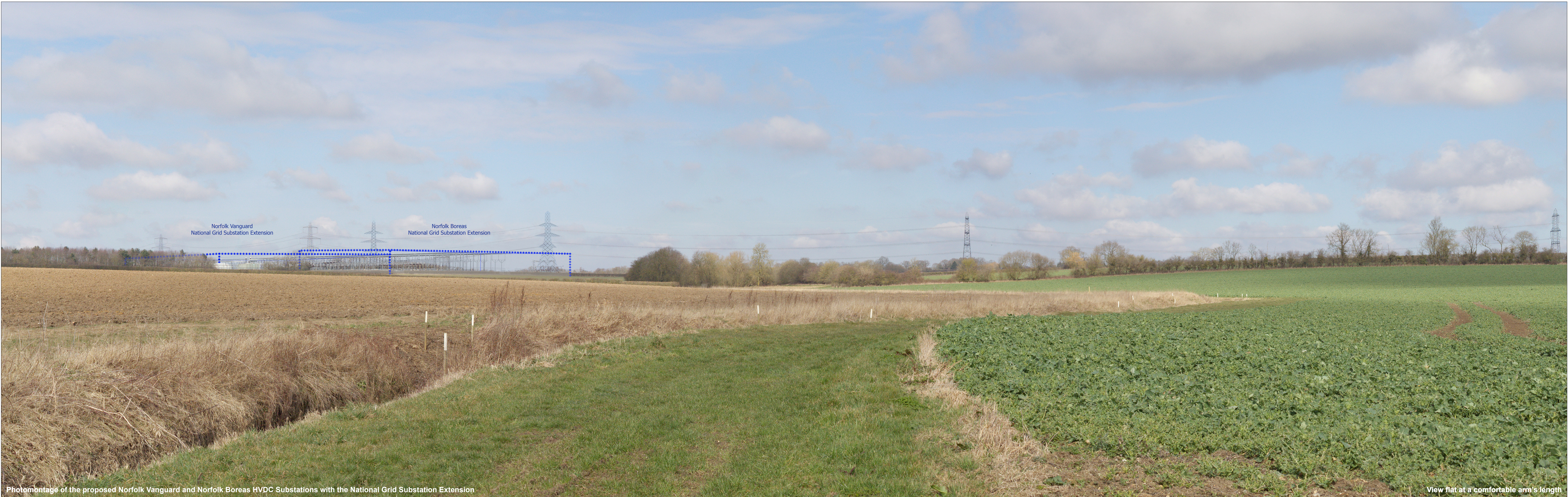
Photomontage of the proposed Norfolk Vanguard and Norfolk Boreas HVDC Substations with the National Grid Substation Extension
